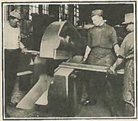
Photo Bridgeport Brass Co. Visual inspection of gate end
