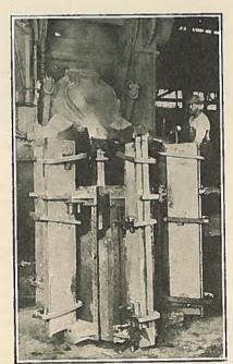
Photo Bridgeport Brass Co. Pouring sheet brass bars
