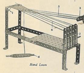
movement of the warp is obtained by moving the Strip 3 up or down, care being taken to see that each thread falls properly between the Strips 2. The shuttle 4-a 3½" Rod—which carries the west, is passed between the two layers of warp 5 and 6
